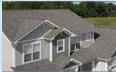
Roofing and Ventilation
